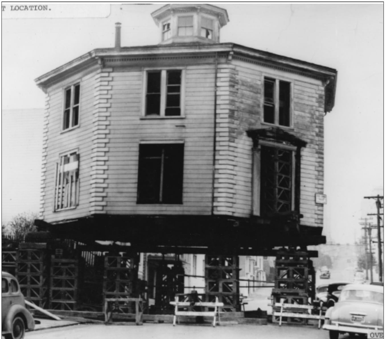
The Octagon House being moved from one side of Gough Street to the other. Courtesy of Octagon House archives.
