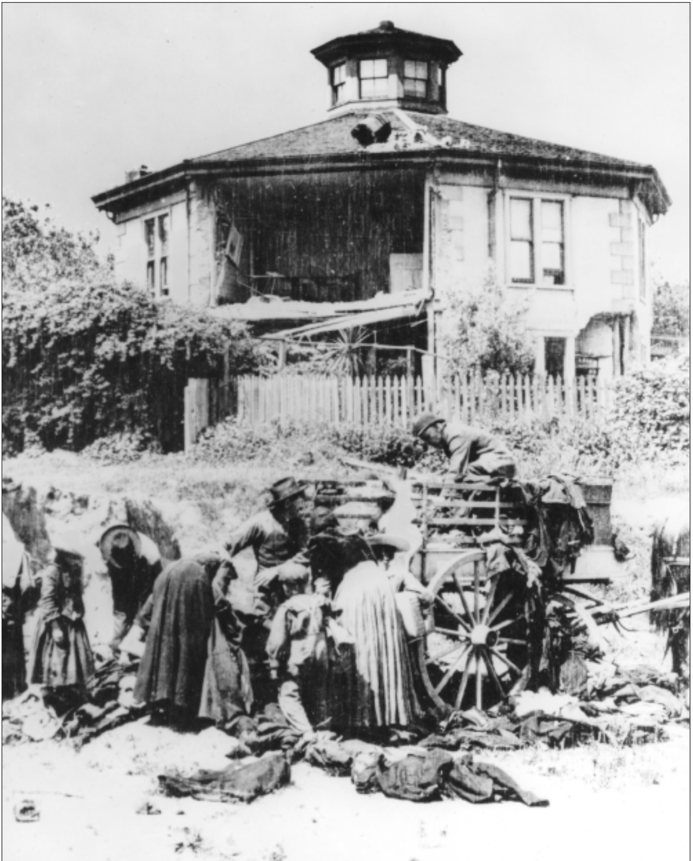
Fiorenzo Cavagnaro, a wine merchant, and his family moved into the Octagon House in 1893. While the house was being repaired, they lived in Oakland, but returned in 1907. Photo of Octagon House after the 1906 earthquake. Courtesy of Octagon House archives.
